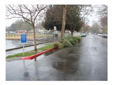
In the picture to the left, note the green waste piled in the gutter. This will often result in an upstream pool of water that extends out into the street and causing a driving hazard.
